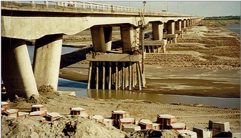
Fig. 1. An example of bridge scour [22]
