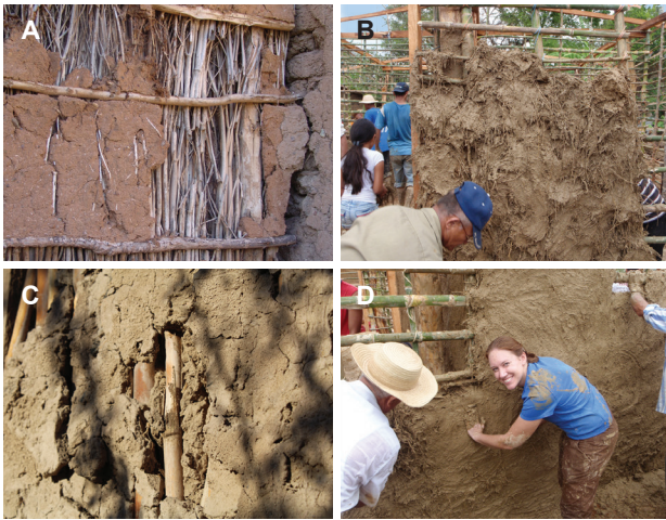
Fig. 5. Contemporary examples of traditional quincha walls (sources: A – https://urbanscrawldc.files.wordpress.com/2014/07/dsc09652.jpg ; B – https://www.revistatierracultah.cl/?p=12501 ; C – https://killpackpanamania.files.wordpress.com/2011/06/p4080190.jpg ; D – https://killpackpanamania.files.wordpress.com/2011/06/p4080227.jpg [accessed: 17.12.2017])
