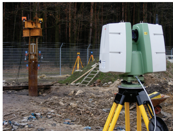
Fig. 1. Application of terrestrial laser scanning to control the vertical displacements during the self-balanced pile capacity testing
