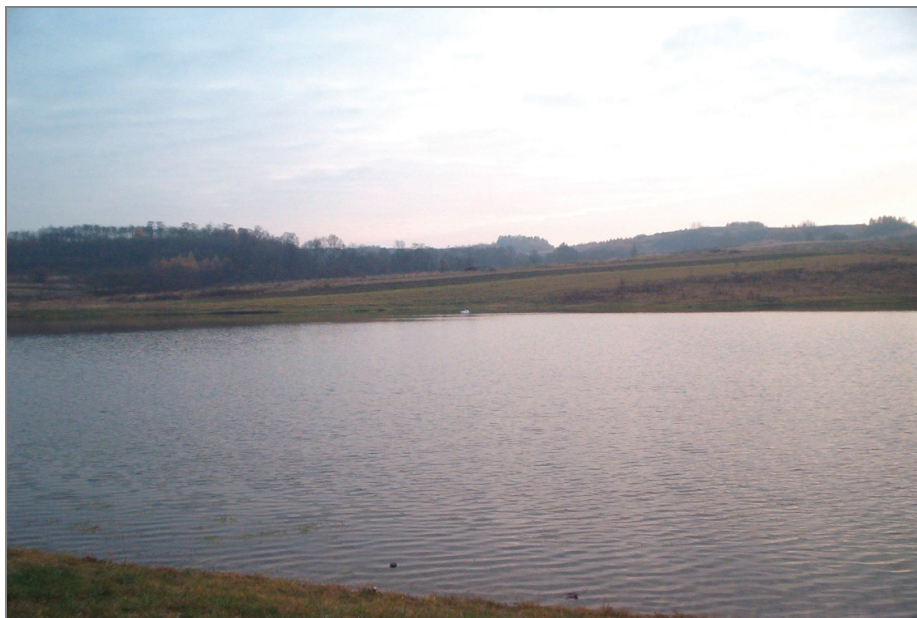
Fig. 3. The existing reservoir in the village of Blizne
