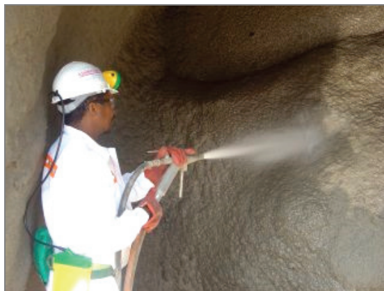
Fig. 14. Typical TSL application (Picture by: Tony White & Associates/Concor)
