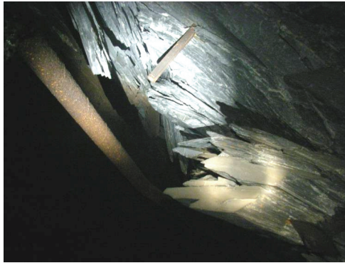
Fig. 6. High stress condition in brittle rock mass
