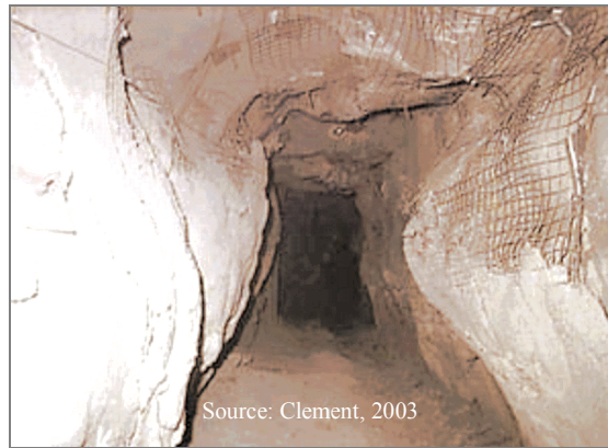
Fig. 11. FRS “Sandwich” to control deformation
