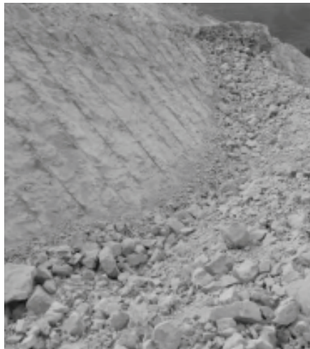
Fig. 9. Smooth blasting effect of roller slope
