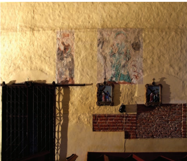
Fig. 2. Photograph of the inner face of the wall in raking light, a base for further analysis (detail of the south wall) (photo: J.M. Arszyńska)
