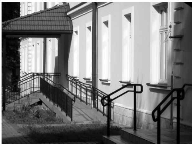
Fig. 9. Adjustment of the school for the needs of the disabled persons (photo: J. Kobylarczyk)
