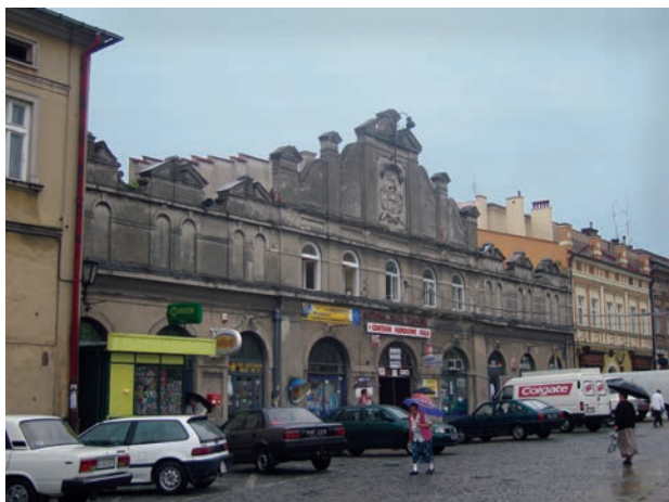
Fig. 2. Market hall – roofed courtyard (photo: J. Kobylarczyk)
