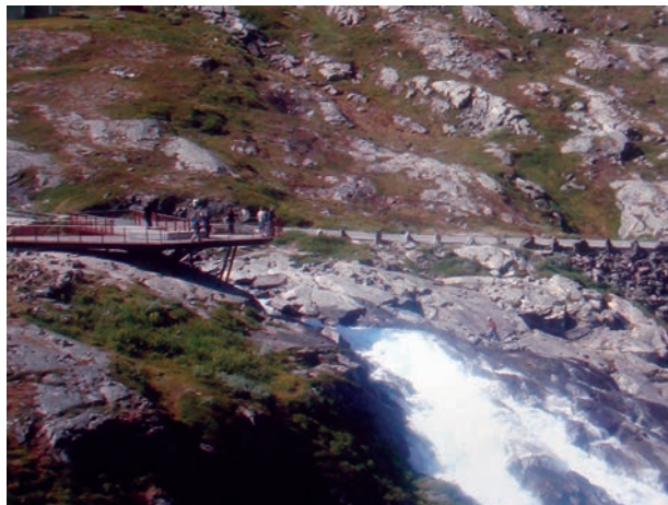
Fig. 1. Trollstigplatået Geiranger – Trollstigen (arch. Reiulf Ramstad Arkitekter AS, under realization 2004–2010) – light steel construction finished with wood enabling observation of Troll Road (photo: E. Cisek)
