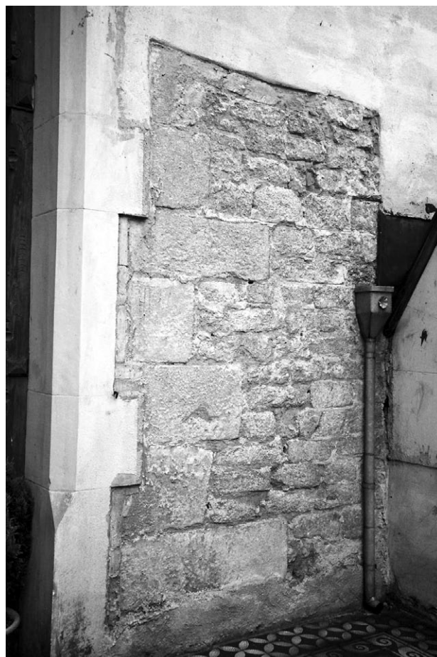
Fig. 8. Corner of the oldest part of south elevation (photo: M. Doroz-Turek)
