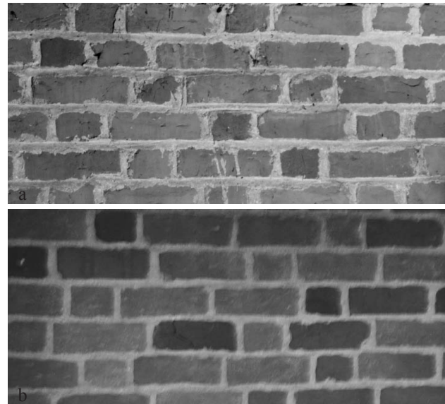
Fig. 7. Brick arrangement in gable between nave and presbytery; fronts: a) eastern, b) western, 2010 (photo: E. Łużyniecka)
