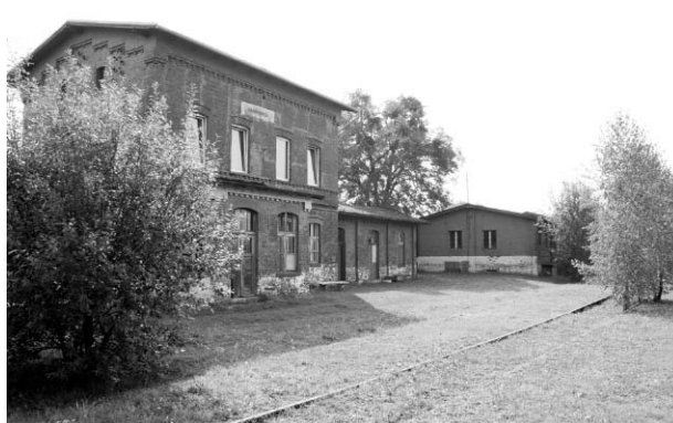
Fig. 3. Krapkowice station. The building is inhabited on the first floor. The ground floor has been unused since 1990. The building is squalid. New and ill-selected window frames in the flat are explicit (photo: M. Konopka, 2009)
