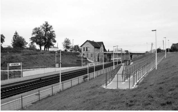
Fig. 10. Łosiów station on the Opole – Wrocław line, rebuilt in 2005–2006 as a passenger stop. Platforms were rebuilt, monumental wheelchair ramps were built, the loading ramp and additional tracks were removed. The building was left unchanged (photo: M. Konopka, 2009)
