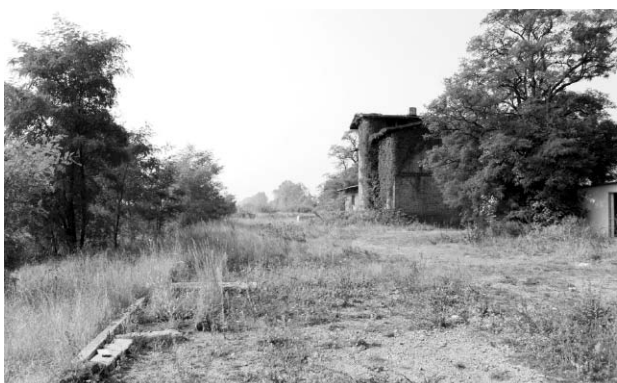
Fig. 8. Łącznik station. Currently the station building is unused. Periodically small wholesale outlets function there (photo: M. Konopka, 2009)
