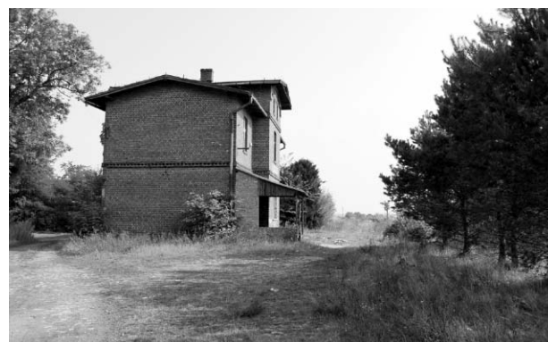
Fig. 9. Strzeleccki station. The building is abandoned and unsecured, and the area around squalid (photo: M. Konopka, 2009)
