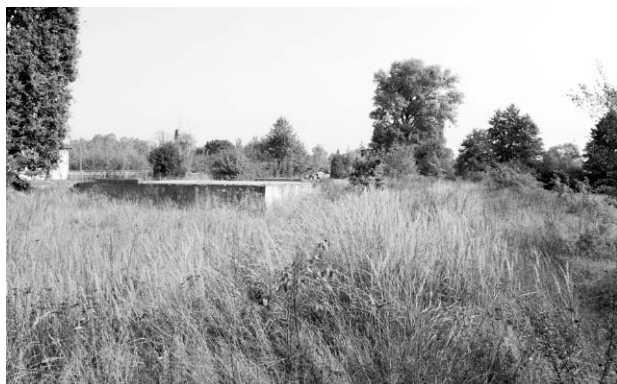
Fig. 6. Zielina station. The station buildings have been torn down. Only fragments of the ramp have remained (photo: M. Konopka, 2009)
