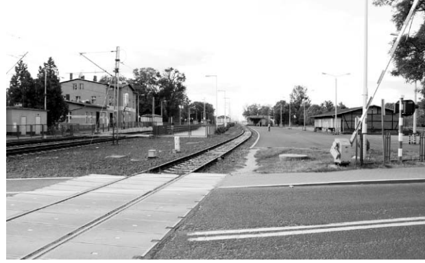
Fig. 11. Lewin Brzeski station on the Opole–Wrocław line, rebuilt in 2005–2006. Platforms were rebuilt, the network of tracks was reorganised, the signal box was reduced to the role of a level crossing attendant's post. The station building was renovated inside and the elevation was rebuilt. The freight yard was renovated. The warehouse and housing buildings were left unchanged (photo: M. Konopka, 2009)
