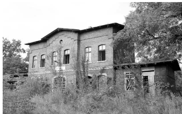
Fig. 7. Biała Prudnicka station. The station is abandoned and squalid. In comparison with other stations on this line it boasts richer brick details (photo: M. Konopka, 2009)
