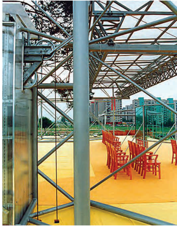
Fig. 10. The papal altar in Sosnowiec, 1999. Steel construction (photo: R. Jurkowski)
