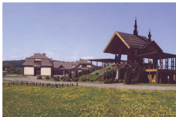
Fig. 12. The papal altar and House of Pilgrim, Stary Sącz. Visualisation. Designed by Z. Remi
