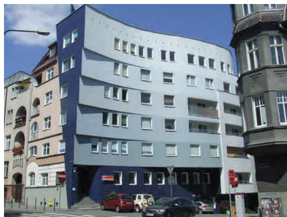
Fig. 5. An in-fill residential building at Kochanowskiego Street 27/28 in Poznań dating back to the 1990s by Klimaszewska & Biedak, an architects. View from the street (photo by A. Nadolny, 2011)
