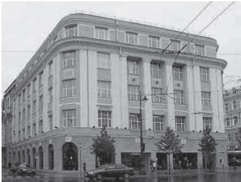
Fig. 1. Vilnius. "Bracia Jabłkowscy" Joint Stock Company Department Store Building, designed by Karol Jankowski and Franciszek Lilpop. Source: [14]
