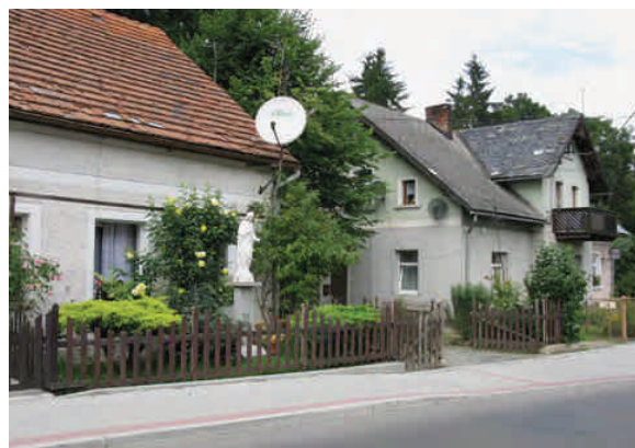
Fig. 5. Houses in Sobieszów (photo by Z. Borcz, 2011)
