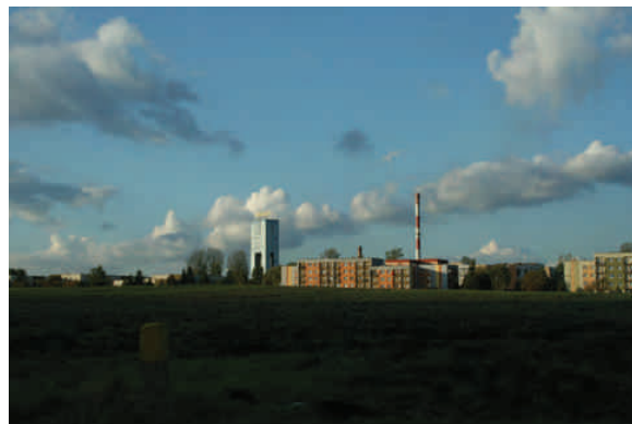
Fig. 11. Multi-family buildings in Bieruń Nowy with "Piaś" mine shaft in the background (photo by I. Niedźwiecka-Filipiak, 2011)
