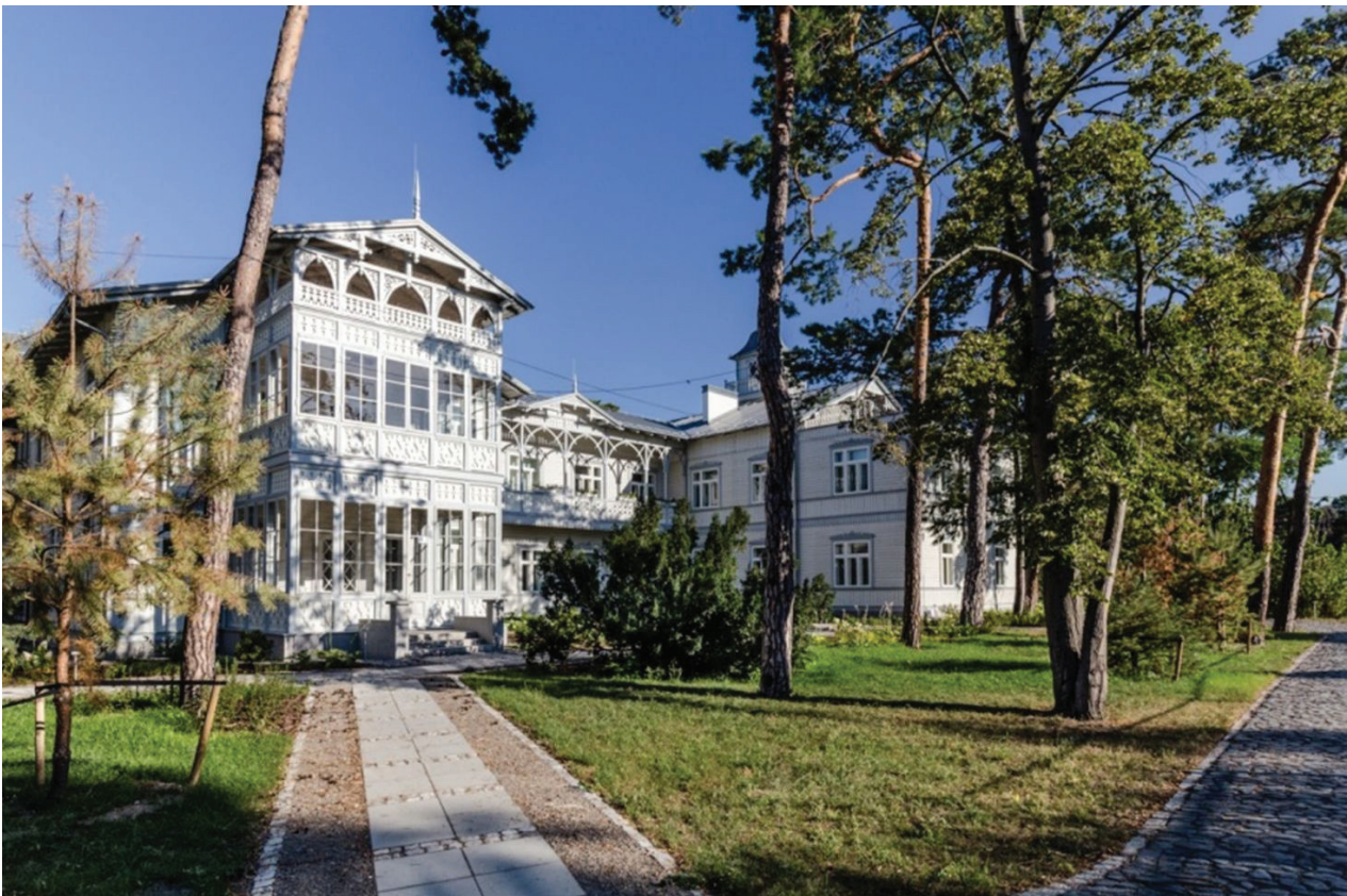
Fig. 10. The wooden veranda of the Abram Gurewicz Health Resort adjacent to the central wing of the eastern façade of the building after its renovation and reassembly (photo by A. Grzesik, the archive of Grupa 5 Architekci)
