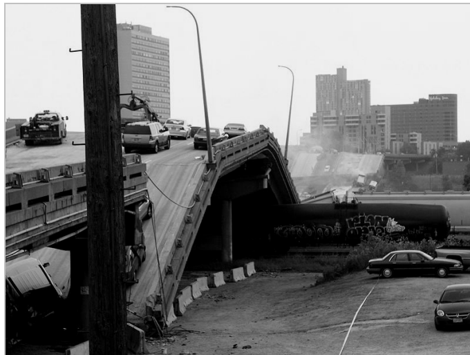
Fig. 2. Collapsed Mississippi River Bridge I35W [3]
