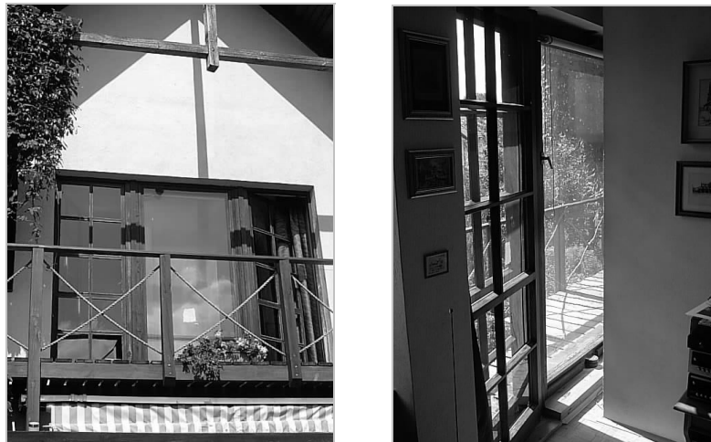
Fig. 11. Hybrid version of the modified CASW, external view on the left side, internal view on the right side
