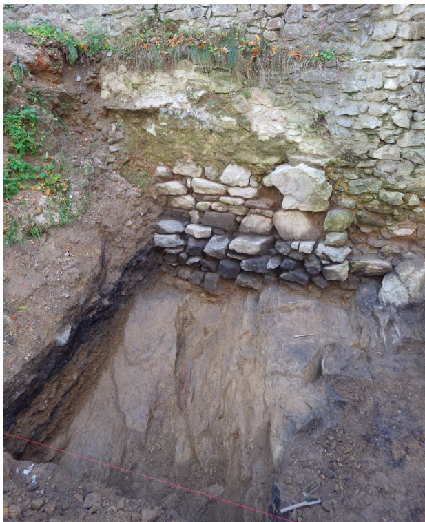
Fig. 3. Probing excavation No. 5 at the wall of the upper castle (photo by Ł. Orlicki)
