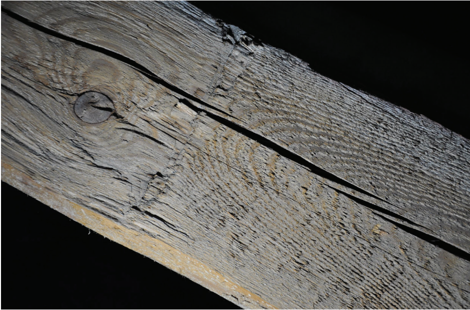
Fig. 12. Leszno, Church of the Holy Cross, roof structure, traces of ax and saw processing (photo by U. Schaaf, M. Prarat)
