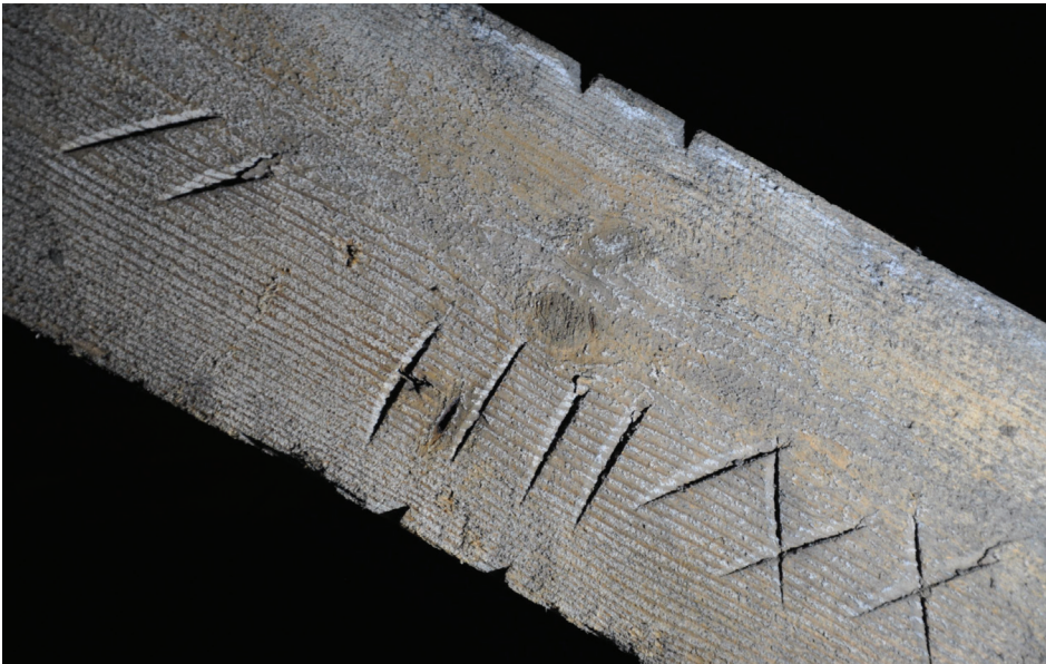
Fig. 13. Leszno, Church of the Holy Cross, roof structure, carpentry assembly marks, Roman numeral in conjunction with by-marks in the form of diagonal cuts and triangular cuts on the edges (photo by U. Schaaf, M. Prarat)
