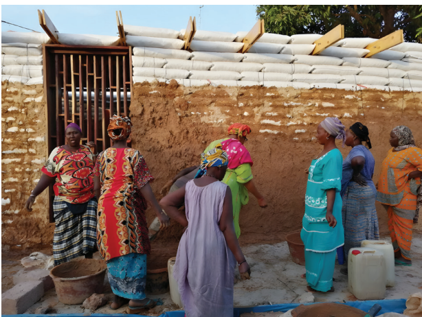
Fig. 2. Polyvalent Cultural Centre, Tanaff, Senegal. Processing of sack walls with earth mortar
