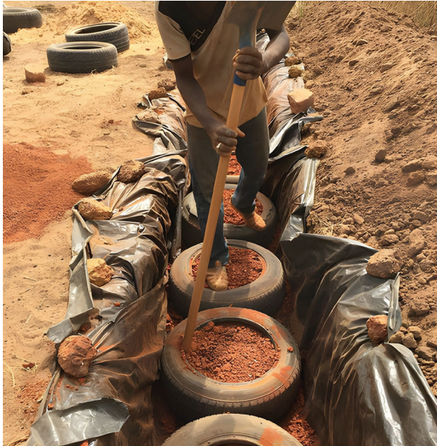
Fig. 5. Primary School, Quartier Dixième, Thiès, Senegal. Foundations made of tires filled with soil (source: image courtesy Let's build my school – humanitarian organization)
