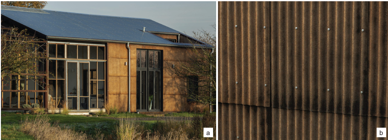
Fig. 9. Zero-emission hemp house Flat House at Margent Farm in Cambridgeshire, England, covered with innovative hemp fiber tiles: a) view of the front elevation, b) detail of the wall (arch.: Practice Architecture, photo by O. Proctor)
