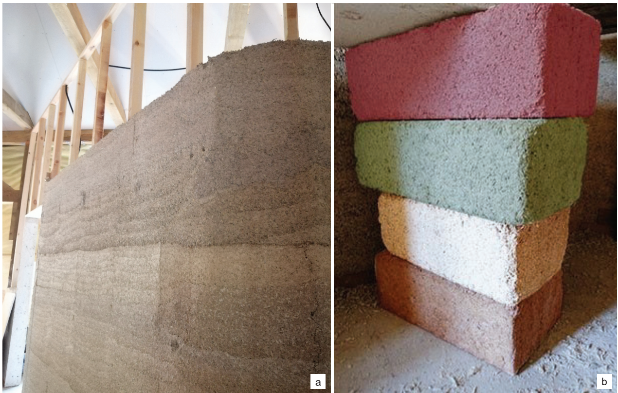
Fig. 8. Various colors, structures and textures of the surfaces of vertical partitions made of hempcrete: a), b) the examples of walls (photo by M. Gacek)
