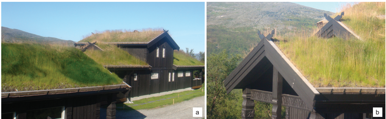
Fig. 1. Extensive green roofs of a residential development in Skaidi, Norway: a) view of the housing development, b) detail: roof with turf-meadow plantings (photo by E. Cisek)
