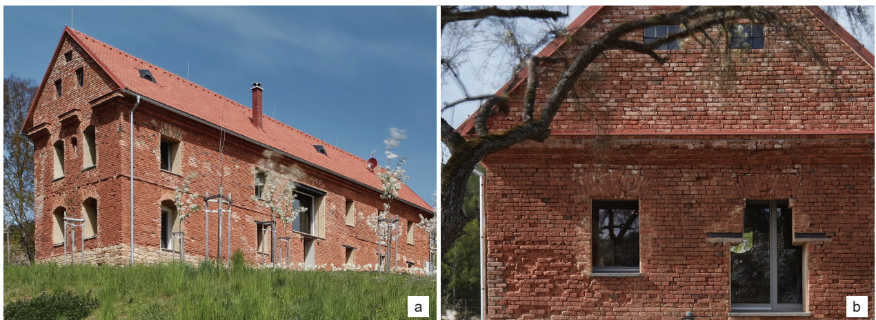
Fig. 6. House inside a ruin in Jevíčko, Czech Republic. The old cottage has become a brick colorful skin for a new home: a) view of the building, b) detail of the brick wall (photo by BoysPlayNice)
