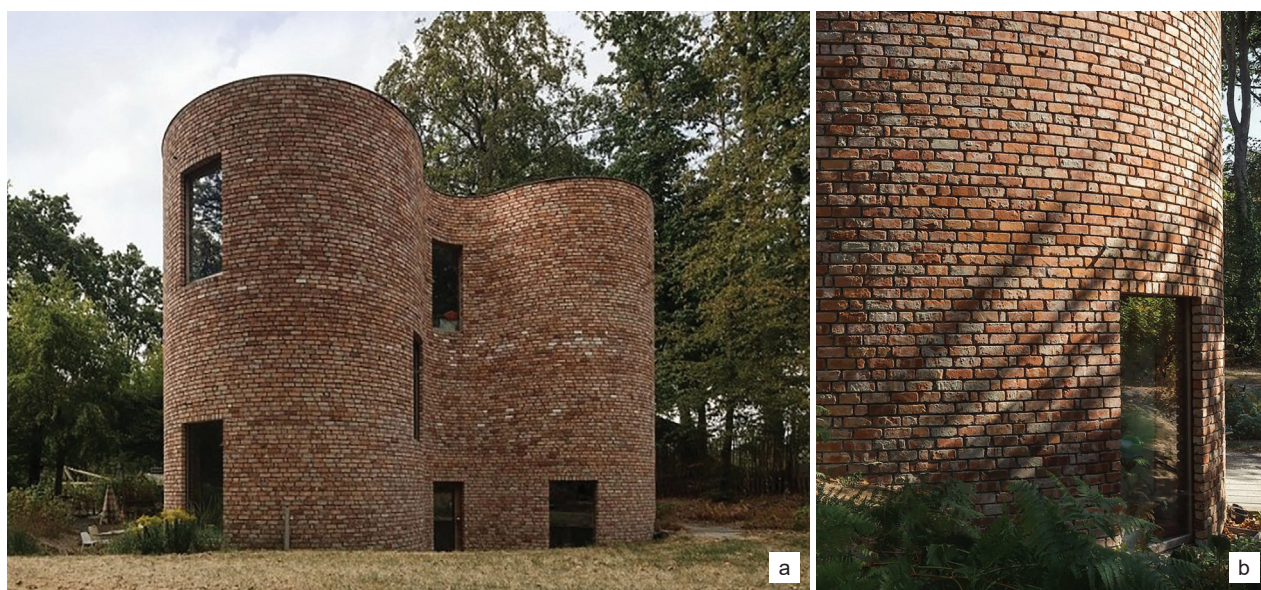
Fig. 4. Unique light and shade transitions of various colors of recycled bricks on the curving surfaces of the walls in GjG House, Belgium: a) view of the GjG House, b) detail of the brick wall (photo by S. Bollaert, BLAF)
