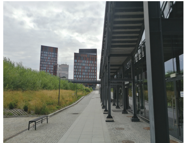
Fig. 7. A cutting along the south wall of the station, originally supposed to admit light to platforms, currently illuminating unused commercial boxes. In the background: “City Gate” office blocks redirected to the axis of Traugutta Street (photo by J. Wesołowski, 2021)
