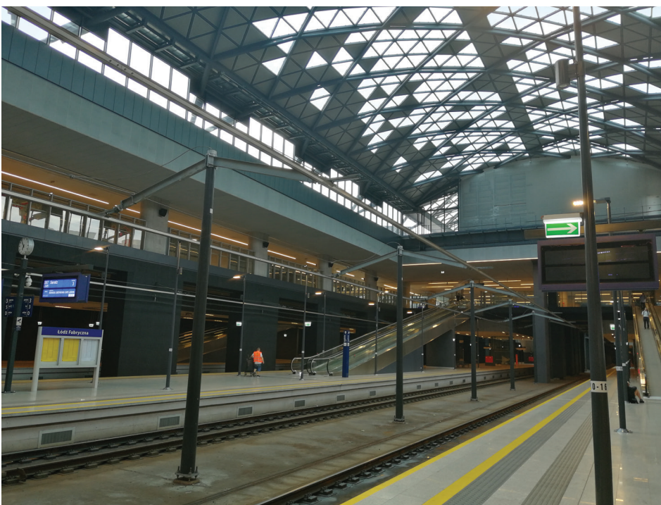
Fig. 6. Middle part of the platforms (level -2) with skylighted overall roofing. Visible is the circulation gallery above one of the extreme platforms (on level -1) (photo by J. Wesolowski, 2021)
