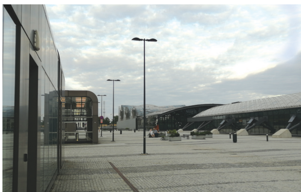
Fig. 11. A vacuum on the north side of the station, awaiting building over. A view towards the middle and rear part of the roofing. To the left: kiosks at the exits from the sub-surface coach station (photo by J. Wesolowski, 2021)
