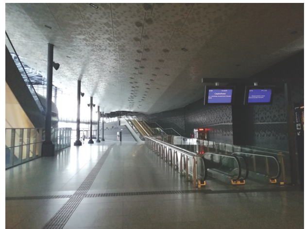
Fig. 13. North gallery. Main exit to tram stops to far right, unintuitive and unmarked (photo by J. Wesołowski, 2021)
