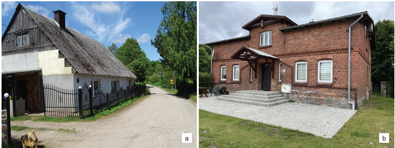
Fig. 2. Two types of farmstead houses in Kashubia: a) a building with a high roof, b) a building with a semi-flat roof (photo by A. Górka)
