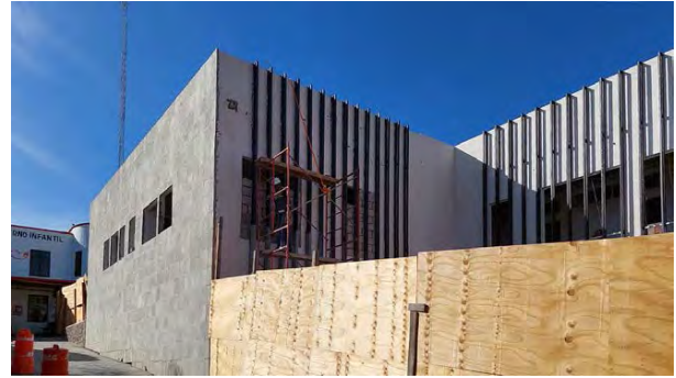
Figure 9: Tepetzotlan Local Public Hospital under construction (2023)
