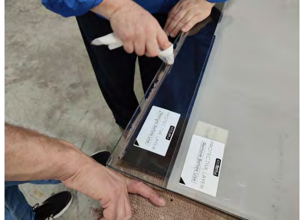
Figure 4: Preparing films for busbar installation.
