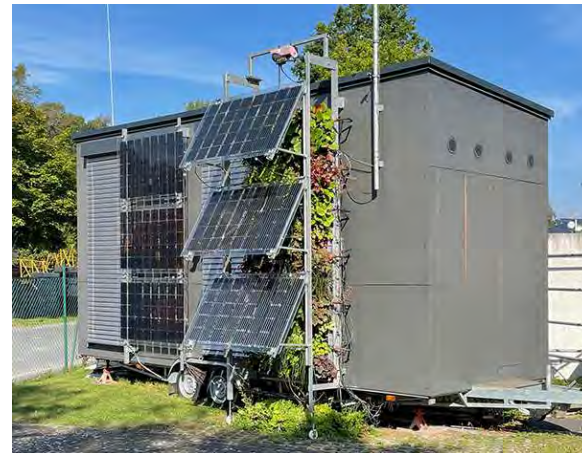
Figure 12: Façade test stand. Reference office with photovoltaic modules (PV) (left) and structure with Kramer greening system / variant 2 and inclined PV modules (30 °) (right) (09/2023)
