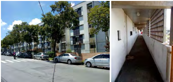
Figures 8 and 9: Architectural elements for shading and natural ventilation of The Corruíras Complex- View of the main facade featuring openings and perforated elements, and view of the common circulation area, emphasizing the use of perforated elements.
