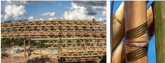
Figure 5: House architecture and 'Group 3+5' connector. Source: Gera Brasil, n.d.
