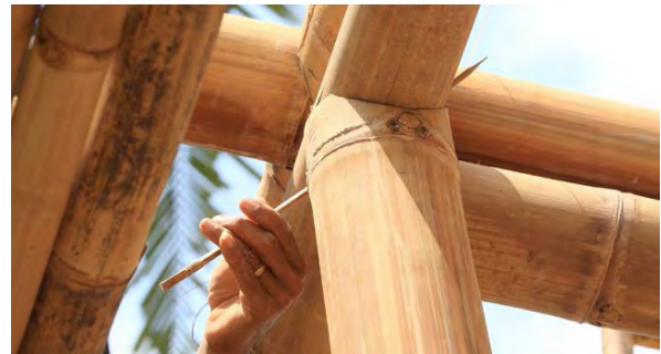
Figure 4: Picture of fish mouth joint with bamboo pin (source: courtesy of Pt. Bamboo Pure)
