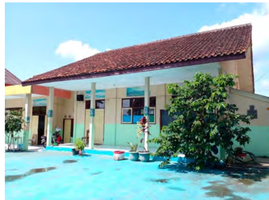
Figure 1: An elementary school building in Jakarta, Indonesia, with clay roof tiles with no insulation. Source: author
