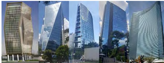
Figure 1 - Photographic survey of geometries: acute and obtuse angular, convex, prism and concave (AUTHOR,2023)
