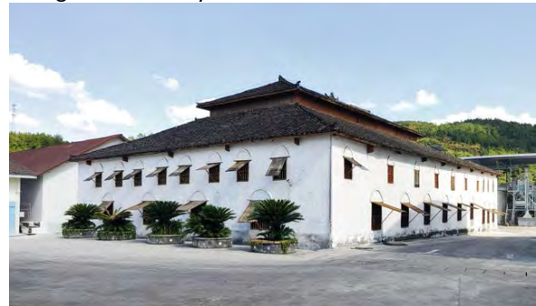
Figure 3: The exterior view of Xuanen No. 1 granary.
