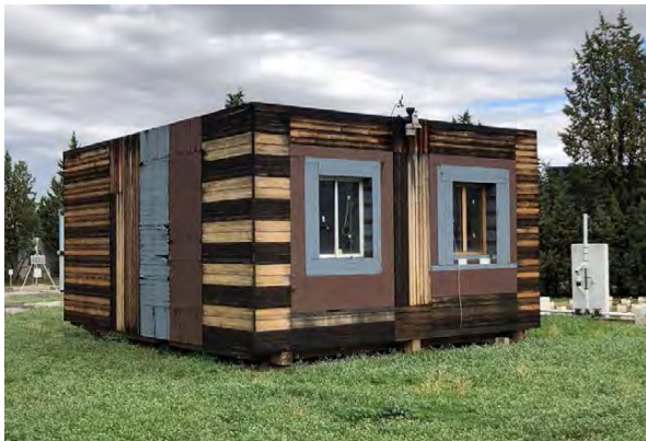
Figure 9: Experimental cells in Arganda del Rey, Madrid, where the prototype of the radiative cooling system of the European PaRaMetriC project will be installed.
