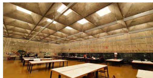
Figure 7: Studio spaces with daylight reintroduced in 2015.
