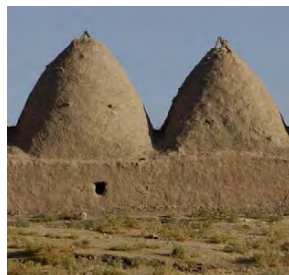
Figure 2: Beehive-like roofs in Harran, Turkey made of limestone. Their profile is identical to the much earlier Assyrian conical domes, due to the same construction technique. Source Wikipedia.
