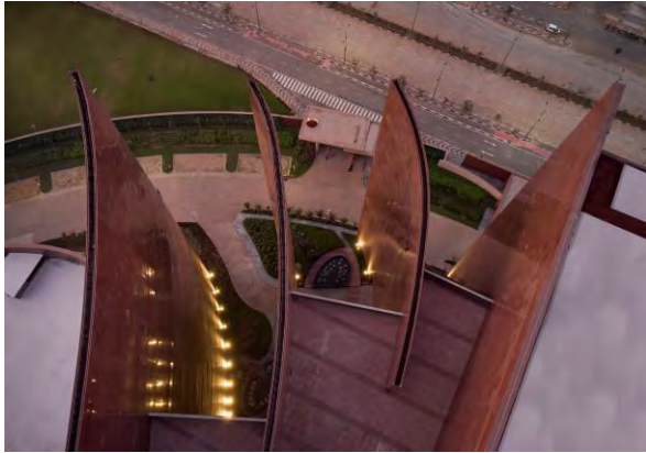
Figure 6: Top view of spine walls – a naturally ventilated, micro-climate tempered community corridor through “Venturi effect”.
