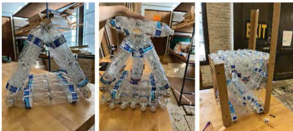
Figure 3: Construction process of a project – utilizing truss structure for the support (source: Omid Elhami, Maryam Sinejani).
