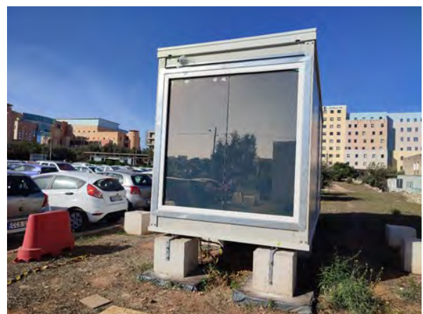
Figure 9: The prototype switchable laminate installed within a test cell.
