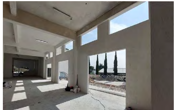
Figure 11: Polideportivo Tepozotlan under construction (2023)
