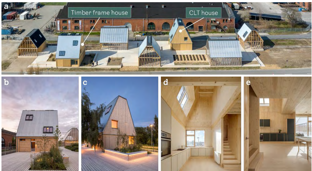
Figure 2: Pictures of the built houses in Living Places Copenhagen. a: Overall view of the area; b and c: Outside view; d: Inside view of the timber frame house; e: Inside view of the CLT house. Photos: Adam Mørk
