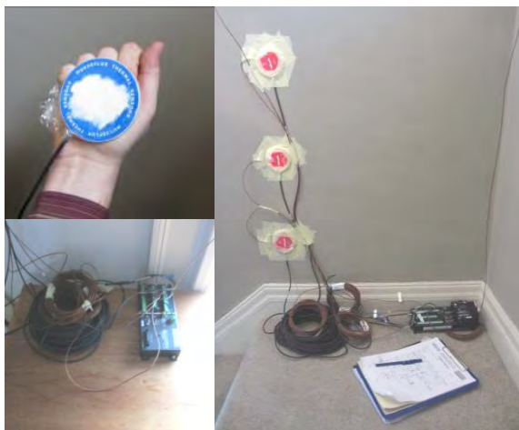
Figure 2. Built to Last heat flow meters, thermal couples data logger and set up.
