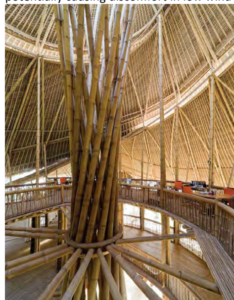
Figure 12: Permeable hyperbolic structural core
