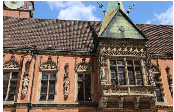
Figure 1: Wrocław Townhall after renovation (2003). Authors
