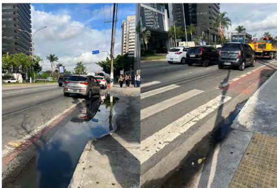
Figure 6: Photographic registers of the rain puddles from the on-site visit.
