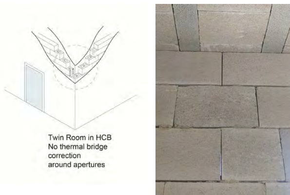
a) Figure 4: The full-scale test cell reproduced from [7]. a) DCB and b) the wall to roof junction showing the evident absence of homogenous mortar joint in vertical and horizontal directions.
