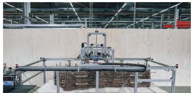
Figure 6: Digital prefabrication of willow structures as scalable construction technology based on initial student work and subsequent development within interdisciplinary research.
