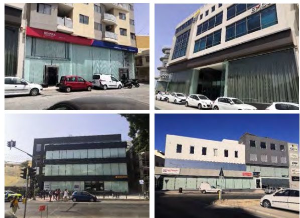
Figure 1: Buildings with a high glazing ratio in Malta, relying on indoor blinds for the control of glare.
