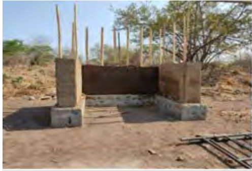
Figure 3: Experimental Rammed Earth Module.
