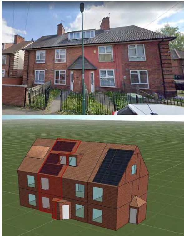
Figure 1: Mid-terrace house (Top) from Google Map data (2023) and simulation model (Bottom)
