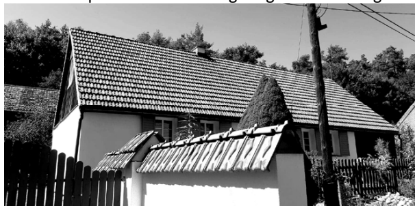
Figure 10: The building after rebuilding, source: author
