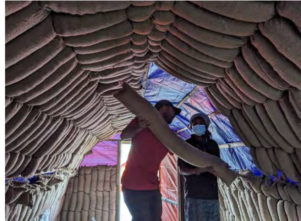
Figure 6: Rice husk packed into jute tubes to act as insulation for a prototype temporary shelter for earthquake victims. Source: Author
