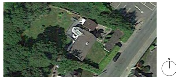
Figure 6. Aerial view of Case Study 1, Google Maps.
