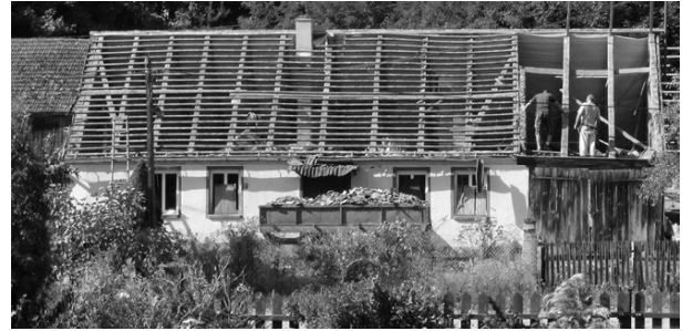
Figure 2: Building before renovation, source: M. Okła
