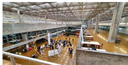
Figure 5: Overview of Salão Caramelo, showing the overarching roof with the field of skylights and the vision communication among the internal spaces below it, qualified by daylight.
