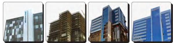
Figure 1: Intervention on the facade of a building in Brasília
