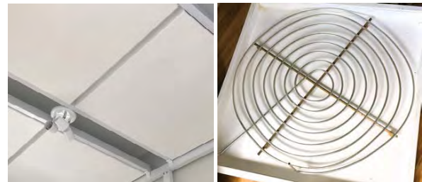
Figure 3: RCMs as ceiling elements and the 3/4" diameter aluminium coil inside the RCM as a heat exchanger.
