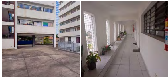
Figures 10 and 11: Architectural elements for shading and natural ventilation of The Jardim Edite Complex- View of the internal facade featuring openings and view of the common circulation area, emphasizing the use of perforated elements.
