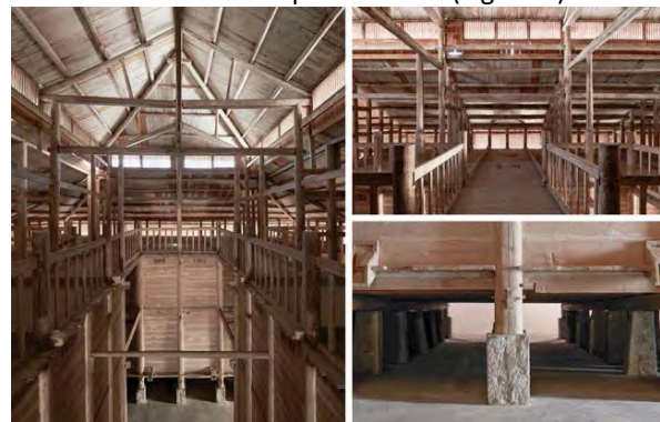
Figure 4: The interior views of Xuanen No. 1 granary.
