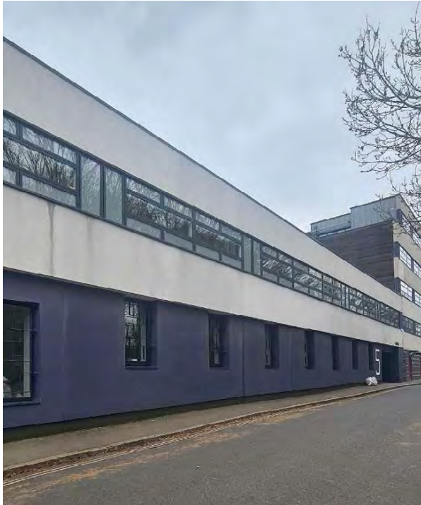
Figure 1: North façade of Cullinan Studio's Foundry Project.
