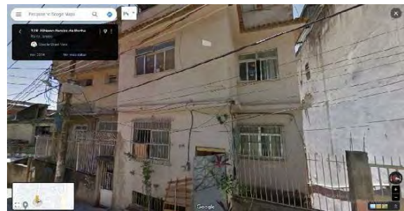
Figure 9: The case-study building. Photo: Google Maps.
