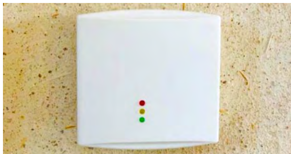
Figure 1: CO 2 sensor with traffic light display in a classroom (Site visit A, 2023)
