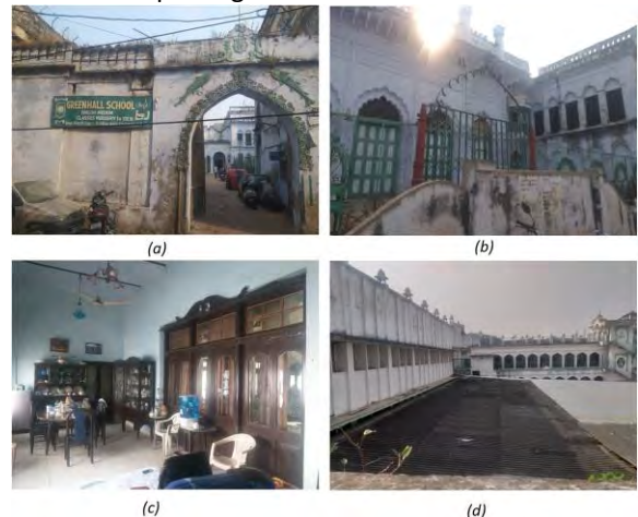
Figure 8: Iqbal Lari Manzil (a- Main Gate with the school board, b- Imambara, c- Verandah converted into Dining Room, d – Garden converted into commercial parking)
