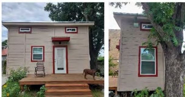
Figure 1: Exterior views of the tiny-house building.
