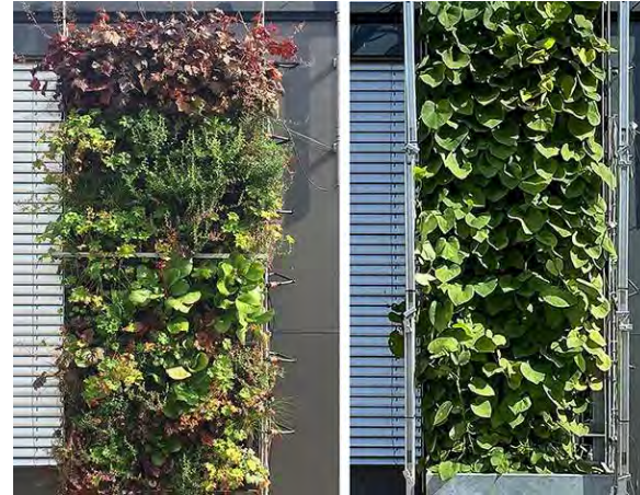
Figure 5: Greening systems: Variant 3 - Kramer Gartenbau, Munich (left / 07/2020) Variant 4 - Jakob GmbH, Ostfildern, with climbing plants (right / 06/2022)
