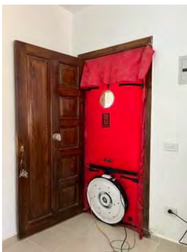
Figure 3: Blower door configuration on tested dwellings.
