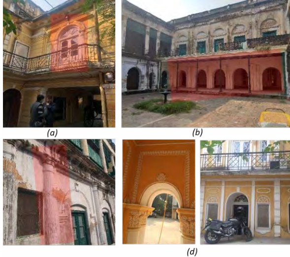
Figure 6:(a- Timber door with semi-circular fanlights, b- Semi-circular arches and multiple entrances on the façade, c- Columns embedded on walls, d – Stucco work)
