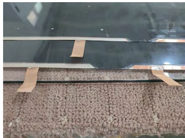
Figure 5: Preparing films for busbar installation.
