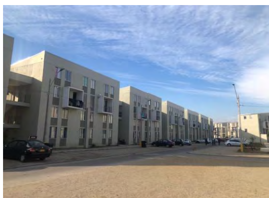
Figure 1: Picture of the apartment buildings of Cordilleras de Doña Marta, Chile.
