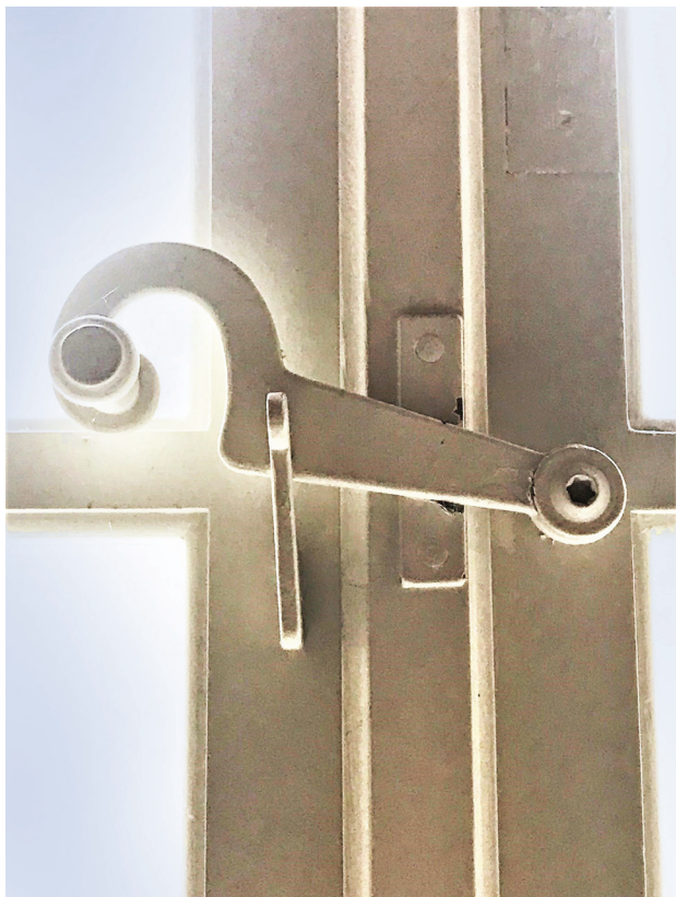
Fig. 3. Cracow, Poselska 7, a deadbolt after renovation (photo by D. Strzałka-Rogal)
