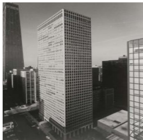
Rys.2.2. DeWitt-Chestnut Apartment Building w Chicago, USA [52]
