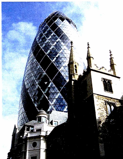
Rys. 94. Swiss Re w Londynie (arch. N. Foster) Fig. 94. Swiss Re in London (designed by N. Foster)
