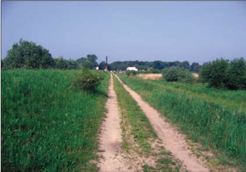
Photo 14. Bench on the embankment used as unsurfaced road
