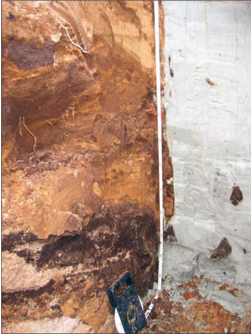
Photo 22. Boundary between the cut-off wall and the soils forming the embankment
