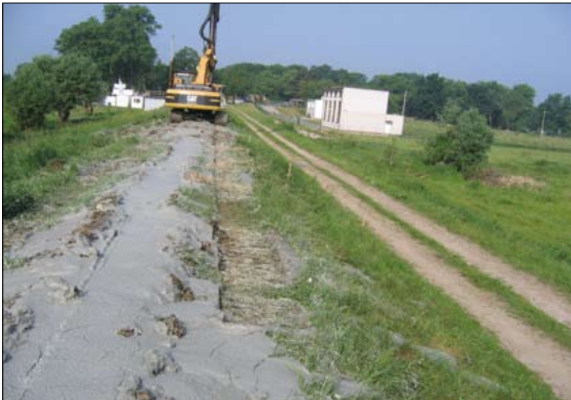
Photo 16. Fragment of the constructed hydraulic cut-off wall
