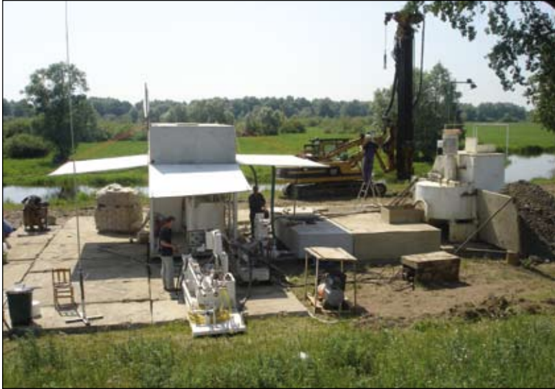
Photo 15. Equipment for the injects preparation, ready for work on the flood bank on Warta in Kostrzyn
