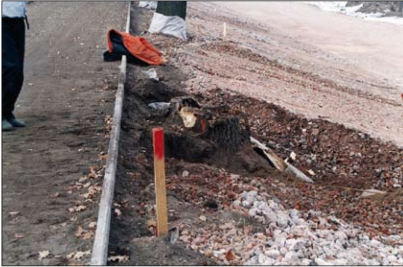
Photo 8. Trees growing on the embankments
