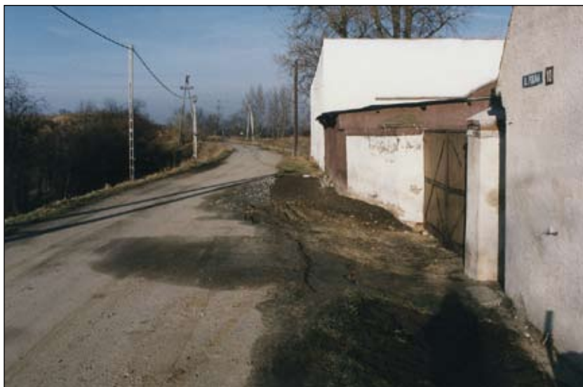
Photo 6. Subsidence of loose soil
