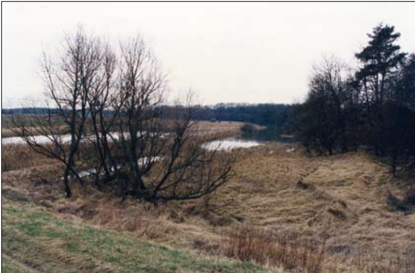
Photo 5. Small ponds of water in the embankment adjacent area
