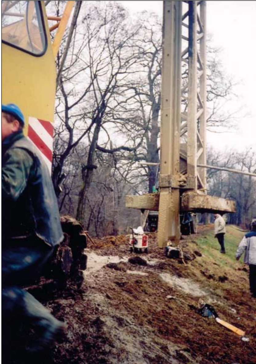
Photo 12. Construction of cut-off wall on the flood banks near Wrocław
