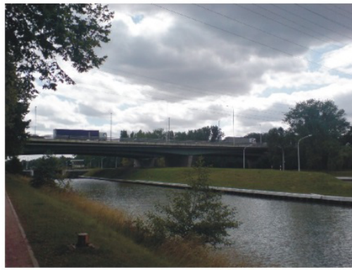
Figure 35: Pictures of the A15 motorway bridge over River Oise in 2008: good structural condition (slab condition of the second bridge on the left – built more recently without tendons – is not so good).
