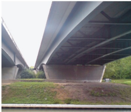
Figure 35: Pictures of the A15 motorway bridge over River Oise in 2008: good structural condition (slab condition of the second bridge on the left – built more recently without tendons – is not so good).
