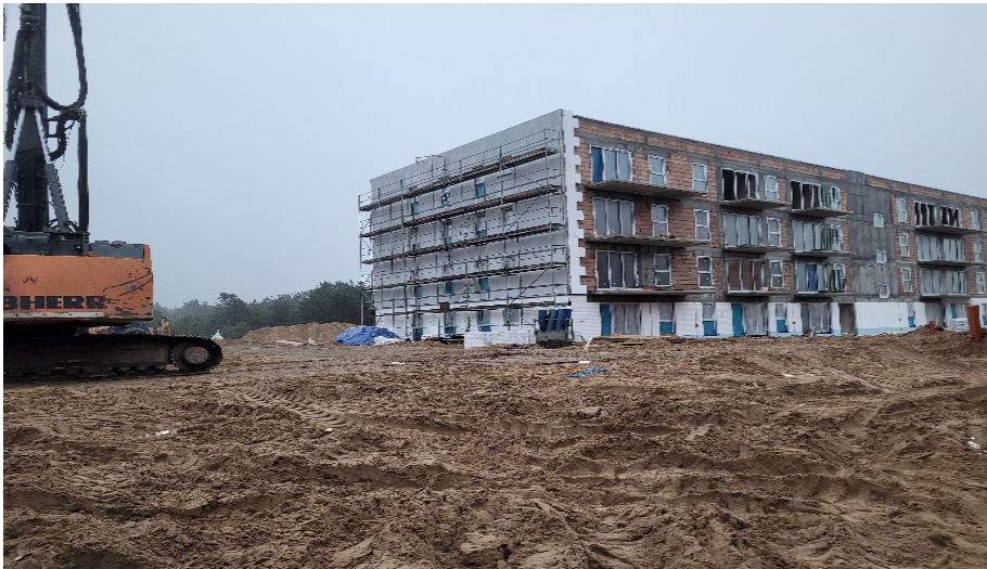
Figure 6: The examined case: vibration-resistant structure located near the soldier pile wall realization.
