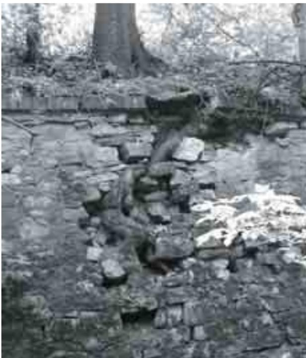
Fig. 17. Destructive influence of plants on the construction structure
