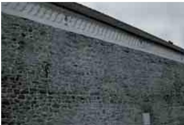
Fig. 9. The west part of the cloister walls from bishop Radziwiłł's time with junction of walls, the so-called toothing, after the preservation in 2008 (photo: O.M. Przybyłowicz)
