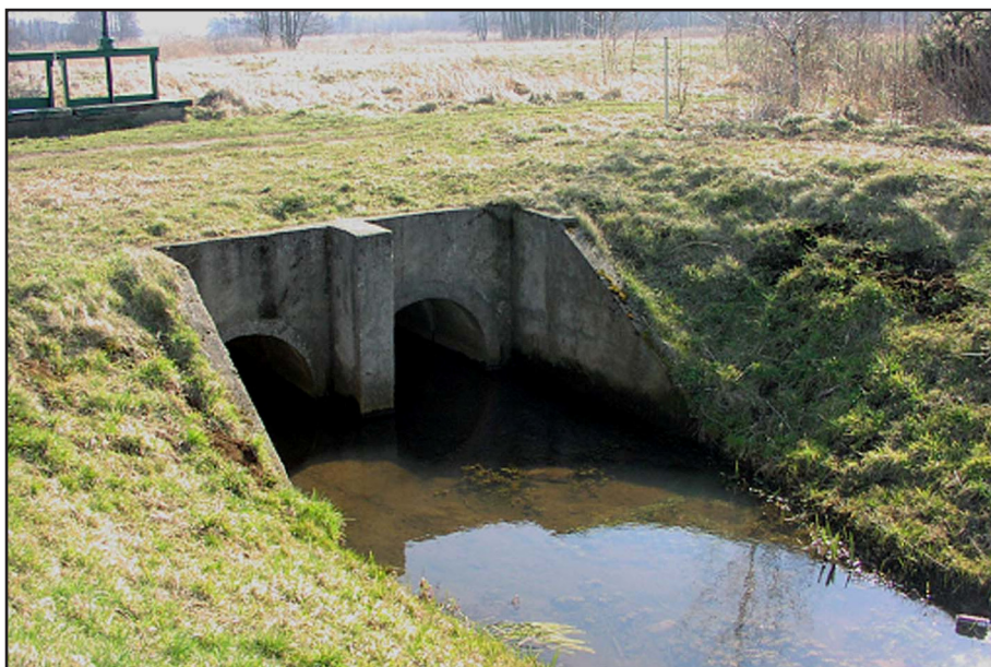
Photo 2. Culvert with damming up on the Zdrojek stream, Miękinia area
