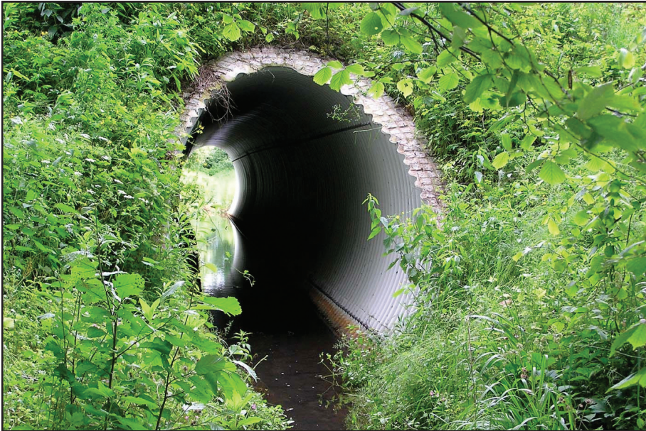
Photo 3. Culvert on the Zdrojek stream
