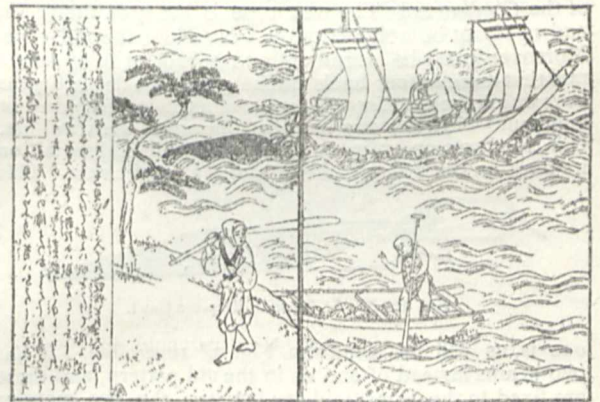
FIG. 1.—Japanese dredge in action.
