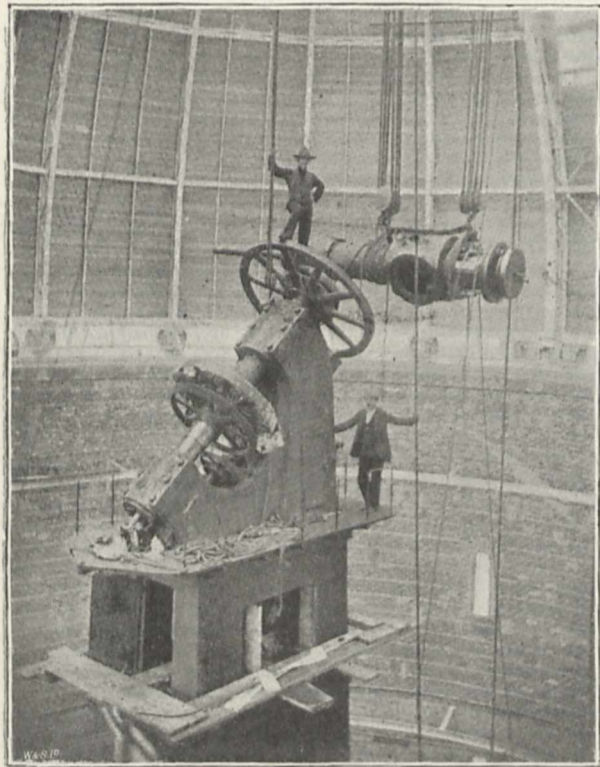
Erecting the declination axis of the Yerkes 40-inch refractor.
