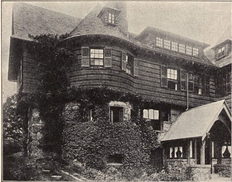
Abb. 877. Haus in Brookline, Massachusetts.
