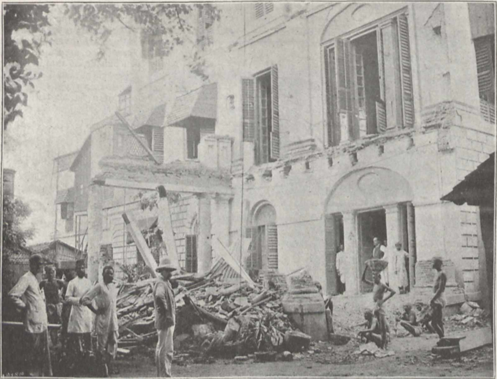
FIG. 1.—Calcutta Earthquake, June 12. Messrs. Traill and Co.'s Office, British Indian Street. A Verandah, with portico beneath it supported on pillars in front of the building, has been entirely destroyed.
