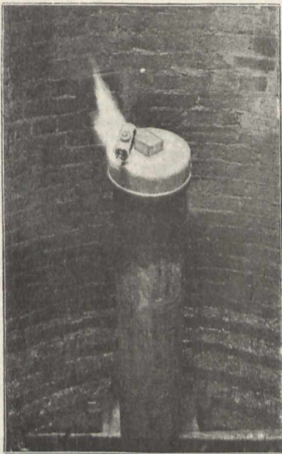
FIG. 2.—Bore-tube in well, with cap having a small vent fixed upon the top. The flame of natural gas is shown rising to the left.
