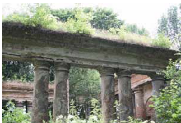
Ryc. 5.160. Zabytkowa pergola, 2008 Fig. 5.160. A historic pergola, 2008
