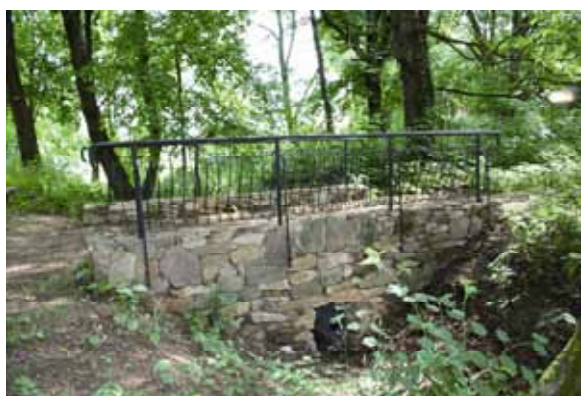
Ryc. 5.159. Odnowiony mostek, 2008 Fig. 5.159. Renovated bridge, 2008
