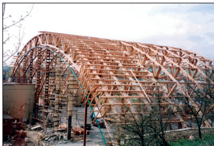
Pic. 1. Roof structure of sports hall in Bílovec
