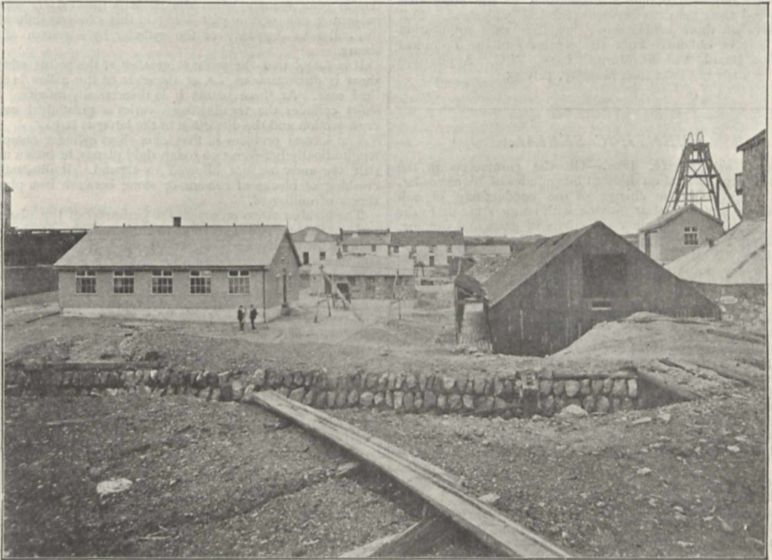
Mine Buildings of Camborne Mining School, Cornwall.
