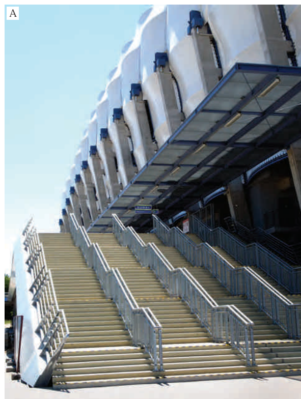
Fig. 6A & 6B. Photos of the façade of the stadium in Poznań. The photo A shows the rhythm of the supporting columns and hopper heads. Below a visible network roofed platform for protection against snow. The photo B shows the rainwater runs. In this case the designer did not design a gutter going along the lower edge, allowing it to drop freely from the edge (photo: M. Pelczarski)
