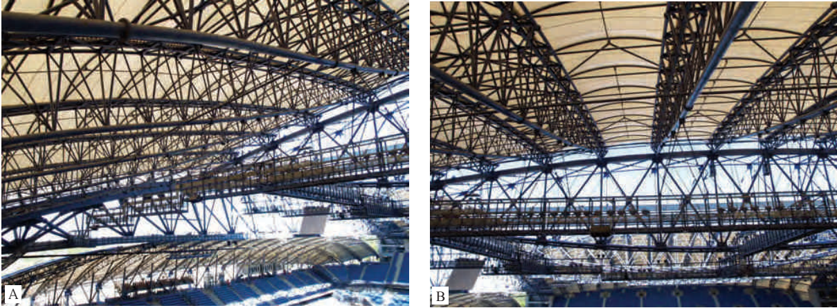
Fig. 4A & 4B. Photos show how the first, second, and third construction planes overlap and cause “an optical chaos”. In such a case the designer must choose whether to expose the aggressive structure to thousands of viewers and present the smooth membrane outside (see Fig. 6A, B) or the other way around. Obviously, extending the construction above the cover exposes it to the elements and their adverse effects and requires a durable anticorrosive protection, but it renders the interior uniform and peaceful. Naturally, the third but costly solution is to apply the membrane under the roof as shown in Fig. 5A, B (photo: M. Pelczarski)
