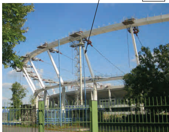
D. Assembly of the roof structure cable-net system in Stadion Śląski
