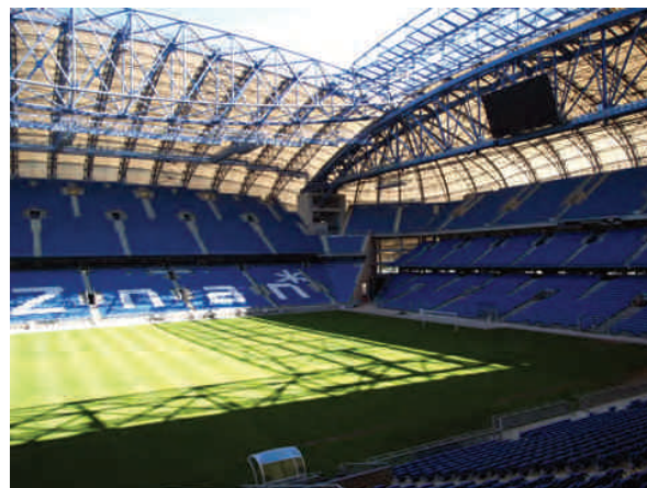
Fig. 3A. Photo of the interior of the stadium in Poznań and the view of the primary 160m long truss with the secondary 135m long, elliptical truss supported on it. The photo shows the “optical ballast” suspended above the heads of thousands of viewers (photo: M. Pelczarski)
