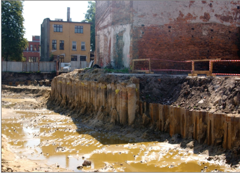
Fig. 2. Pile wall view
