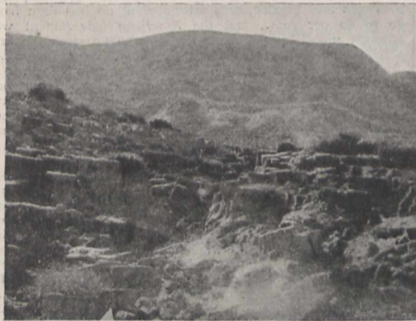
FIG. 1.—Ground disturbed by subsidence, Pallata.
