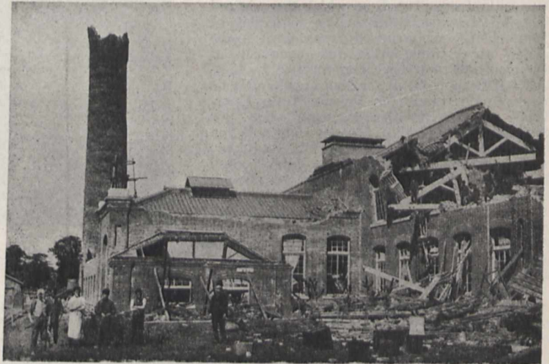
FIG. 2.—Nagoya Spinning Mill. Showing the effects of the Mino-Owari Earthquake of 1901 on a brick building and on a chimney constructed according to European practice.
