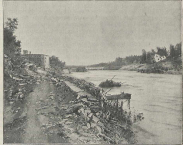
FIG. 2.—Clifton after the flood of 1903.
