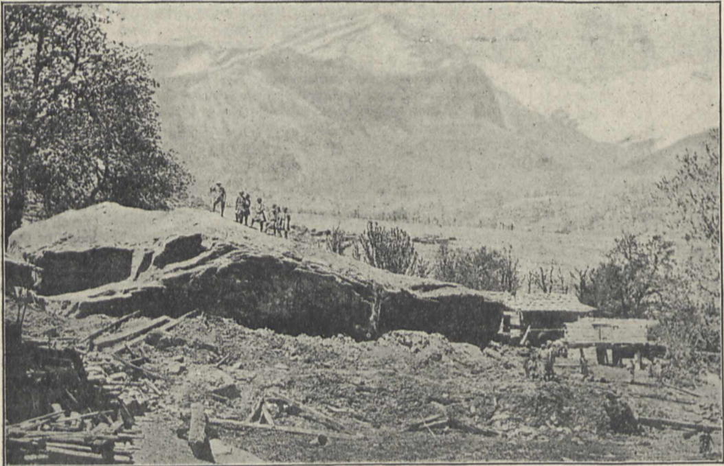
FIG. 1.—Fallen Rock near Manoli. From "The Kangra Earthquake of April 4, 1905."
