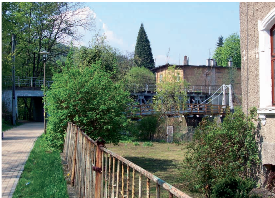
Railway bridge on Biała Głuchołaska among the town buildings – View from northeast
