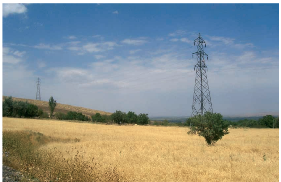
Fig. 8. New infrastructures created new rural landscapes in relationship with the agricultural fields
