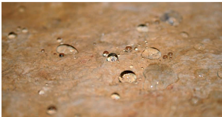
Fig. 5. Water drops at the surface of hydrophobized stone sample
